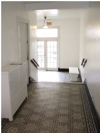
Lobby View to Front Door
